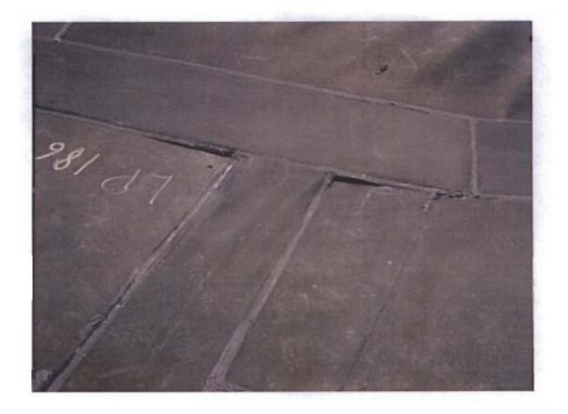
Photo 8: 2007 Seam Defect - Panel 186
