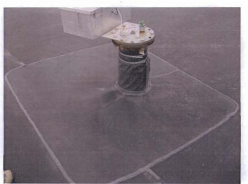
Photo 3: Typical Sump with Liner Boot
