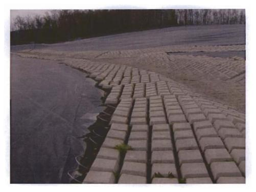
Photo 9: Y-Channel Revetment
